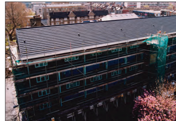
The Slate 2000 can be fixed to timber/steel sub-structures as in this flat to pitch conversion.
