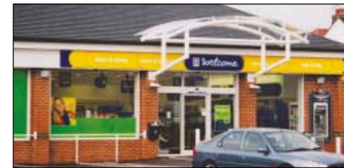
Unlike traditional Slate, the Slate 2000 can be used on roof pitches as low as 12° as well as for vertical hanging.
