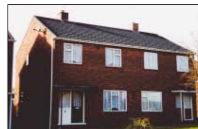
Re-roofing on traditional houses in Slate2000.
