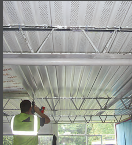
Structural ceiling system
