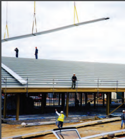
Roofing support system
