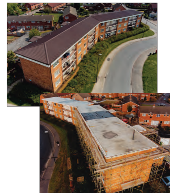
Boldrolls fast-track roofing system considerably reduces time on site, keeping disturbance to a minimum.
