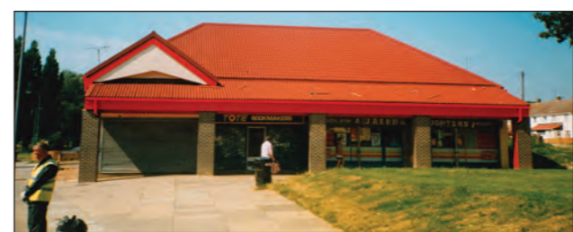
Boldroll ridge to eaves tile effect roofing sheets offer improved structural integrity over traditional materials, making them a popular choice for areas with high levels of vandalism.
